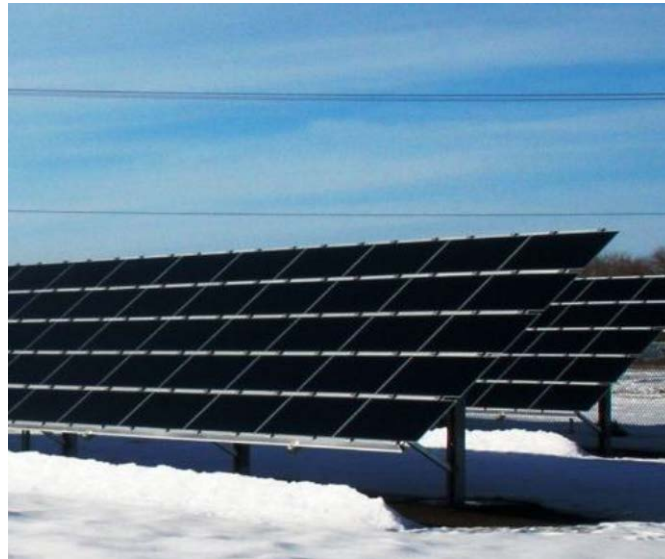
Figure 9.9. Arrays of Thin-Film PV Panels at the Ellensburg Renewable Energy Park (City of Ellensburg 2013a)
