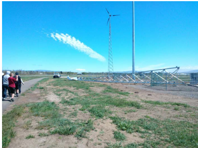
Figure 9.36. Collapsed Tangarie Wind System
