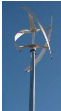
Figure 9.39. 4 kW Urban Green Energy Wind System at the Ellensburg Renewable Energy Park (City of Ellensburg 2013a)
