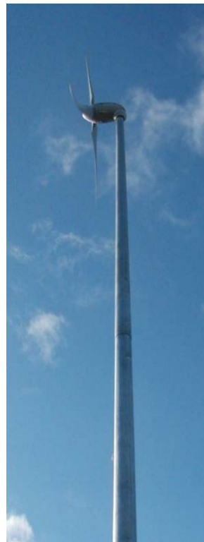
Figure 9.25. 2.4 kW Skystream Wind System at the Ellensburg Renewable Energy Park (City of Ellensburg 2013a)
