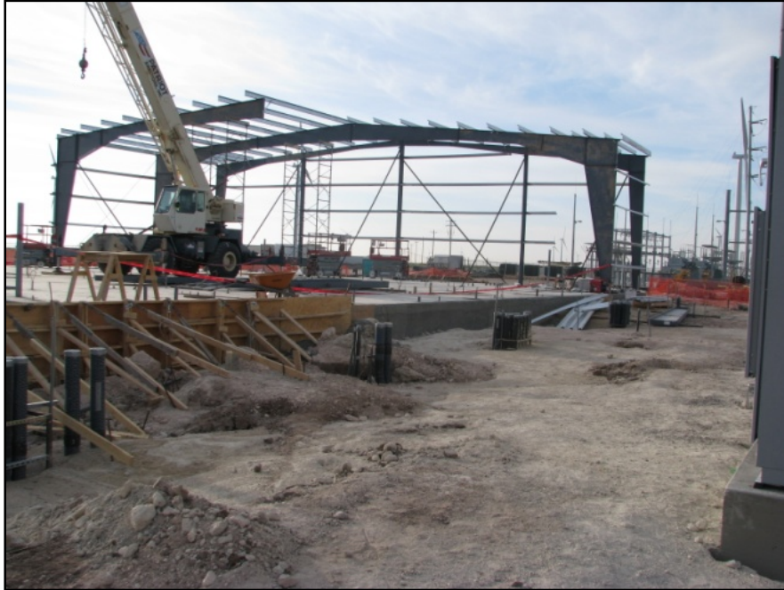
Figure 6-4 Construction in progress
