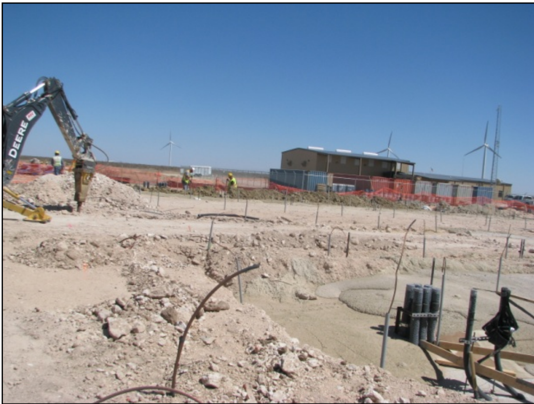
Figure 6-1 Preparations for pouring concrete (view northwest to southeast)
