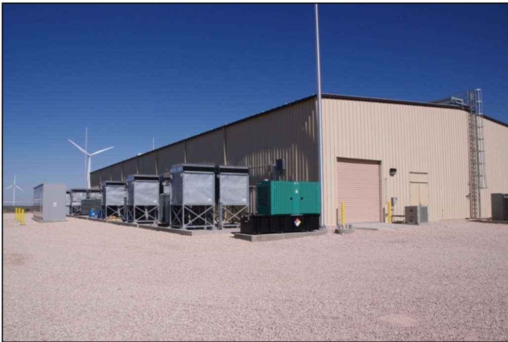
Figure 6-9 Completed building exterior
