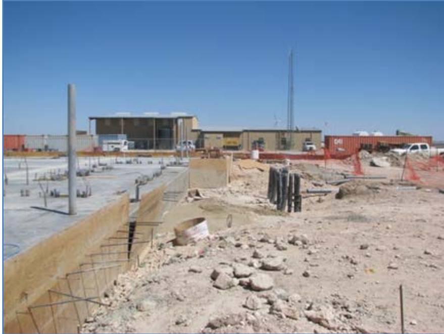
Figure 6-2 Concrete work in progress (view southwest to east)
