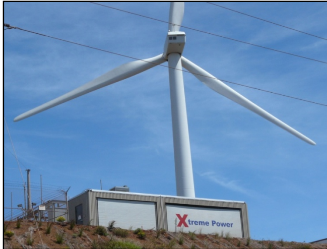
Figure 2-1 1.5-MW/1-MWh Kaheawa Wind Power Project in Maui, Hawaii
