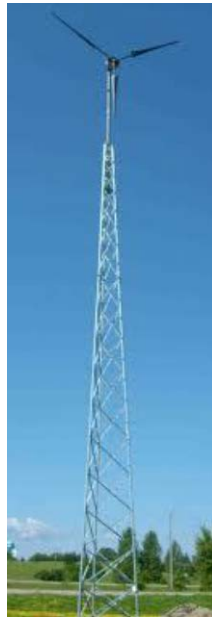
Figure 9.43. 10 kW Ventura Wind System at the Ellensburg Renewable Energy Park (City of Ellensburg 2013a)
