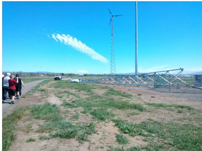
Figure 9.36. Collapsed Tangarie Wind System
