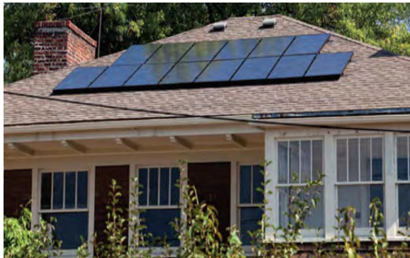
Figure 3-17: Rooftop PV Installation on Project Living Proof Demonstration House
