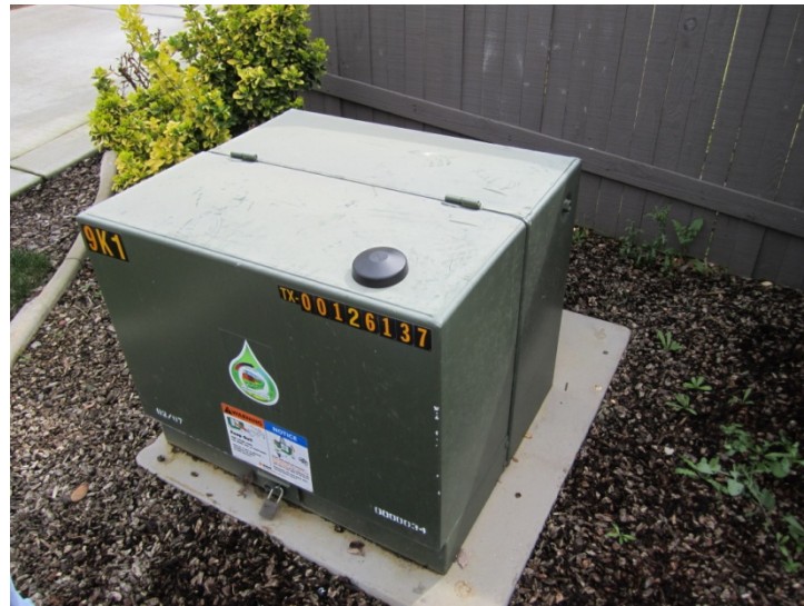
Meter installation on a Pad Mount Residential Transformer in Sacramento %
