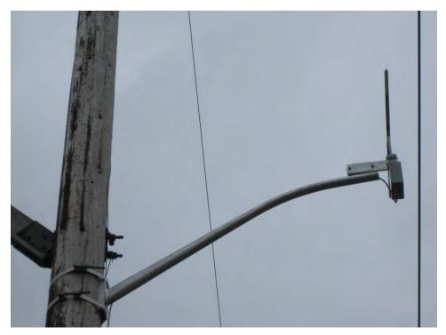
Figure C-67 ThermalRate Sensor and Arm Installed
