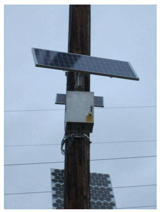
Figure C-63 Sagometer Electronics Box and Solar Panel Installed
