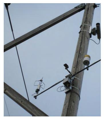
Figure D-3 Weather Station Installation at Site 3
