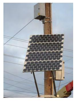
Figure C-68 ThermalRate Solar Panel Installed
