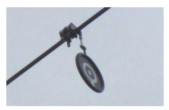
Figure C-69 Sagometer Target Installed
