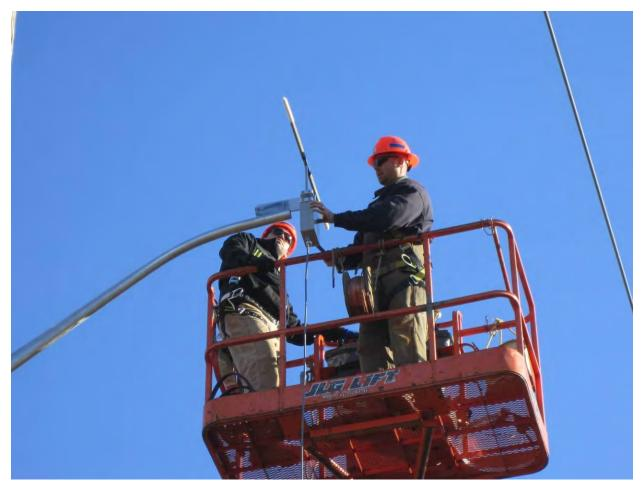
Figure C-45 ThermalRate sensor being installed
