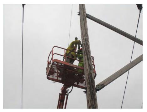
Figure C-60 Installed the Sagometer Camera
