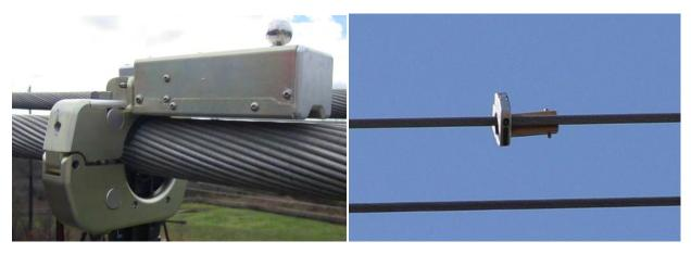
Figure 3-3 EPRI Sensor mounted on a conductor
