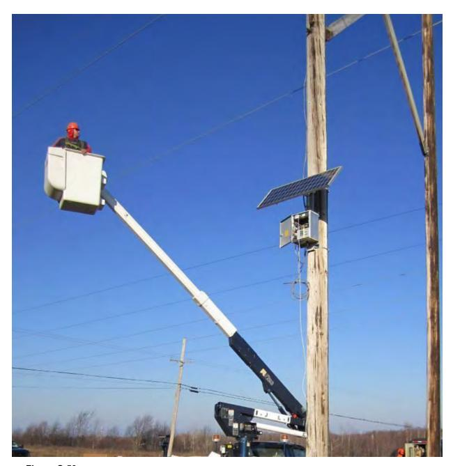
Figure C-50 Sagometer Electronic Box and Solar Panel Being Checked After Installation
