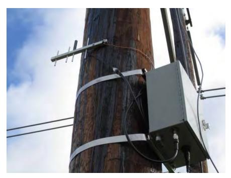
Figure C-34 ThermalRate electronics box and antenna
