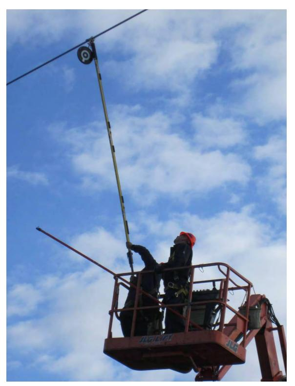
Figure C-49 Sagometer Target Being Installed
