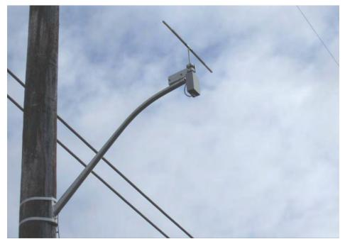
Figure C-33 ThermalRate sensor installed
