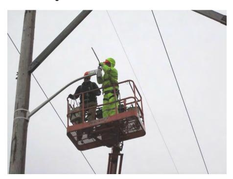
Figure C-57 Installing the ThermalRate Sensor
