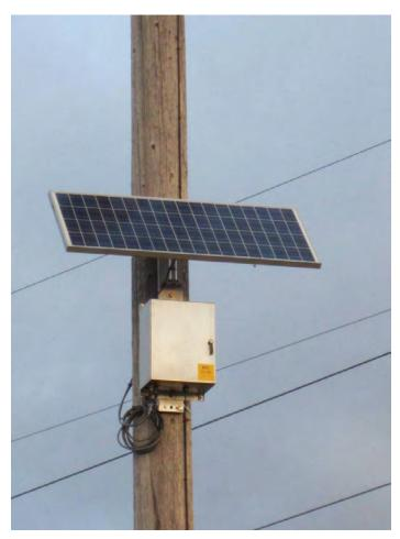
Figure C-70 Sagometer Solar Panel and Electronics Box
