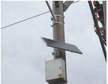
Figure C-66 EPRI Sensor Electronics Box and Solar Panel
