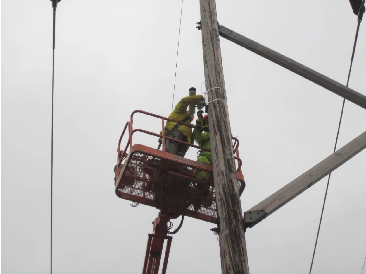
Figure 4-46 Installing the Sagometer camera
