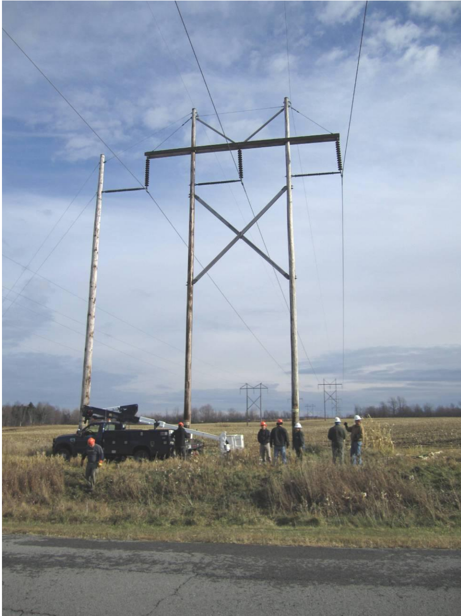
Figure 4-18 A tailgate meeting was held before work begins at WP2-01/02
