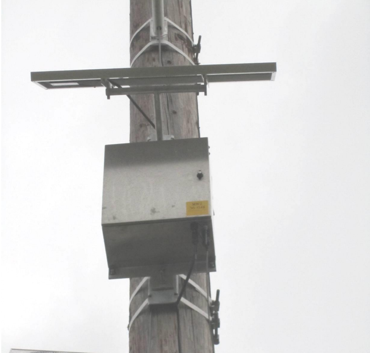
Figure 4-41 EPRI sensor electronics box and solar panel installed
