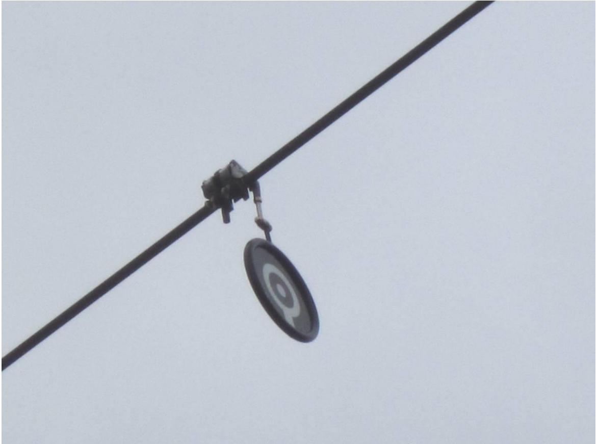
Figure 4-65 Sagometer target installed
