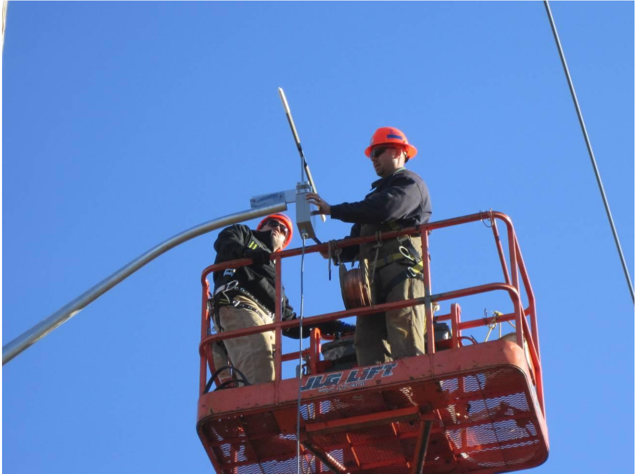
Figure 4-24 ThermalRate sensor being installed
