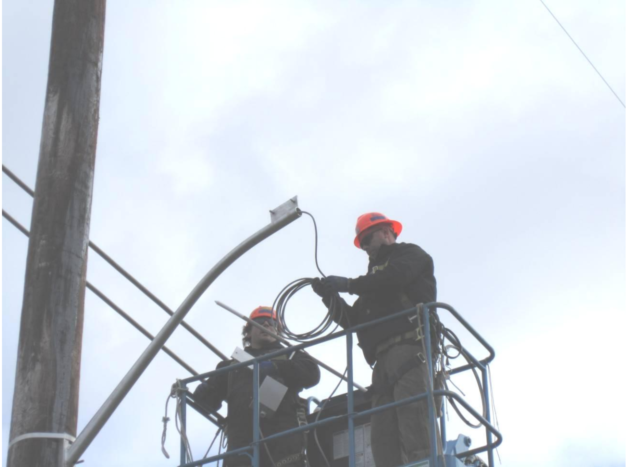
Figure 4-7 ThermalRate sensor being prepared for mounting
