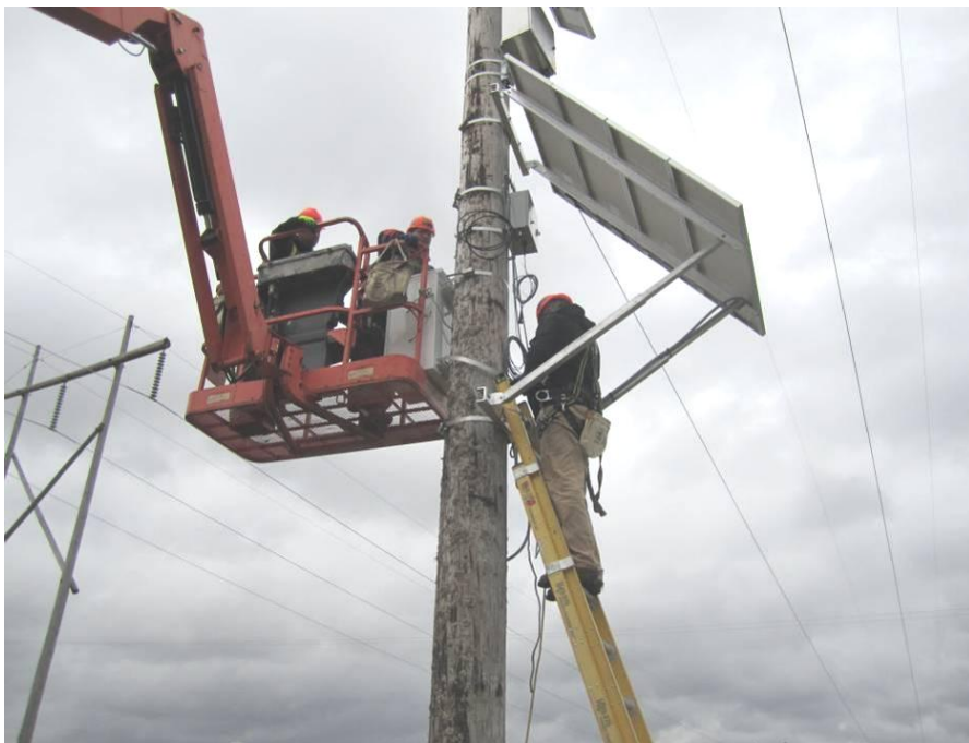
Figure 4-44 ThermalRate system solar panel and electrical box being installed
