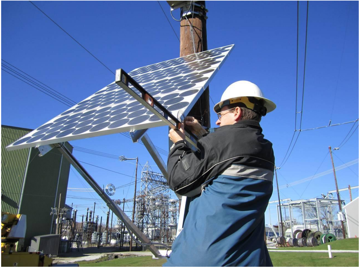
Figure 3-33 Photo of solar System
