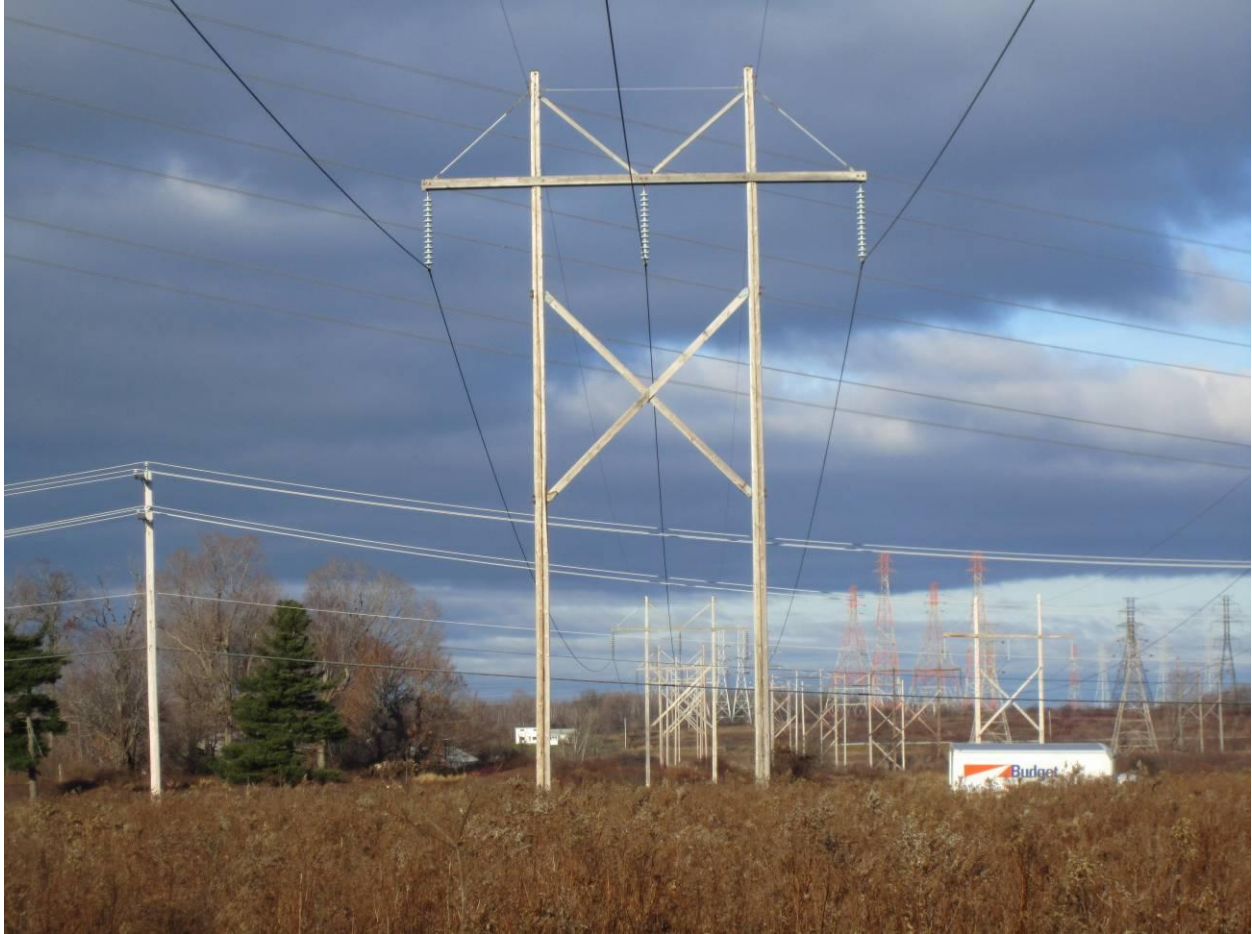
Figure 4-56 Looking back at structure MW2 - 03/06 towards Moses substation before installation begins
