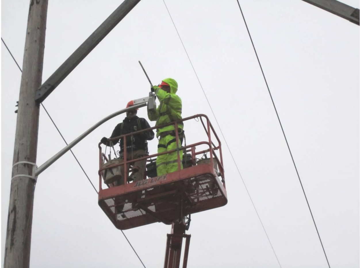
Figure 4-43 Installing ThermalRate sensor
