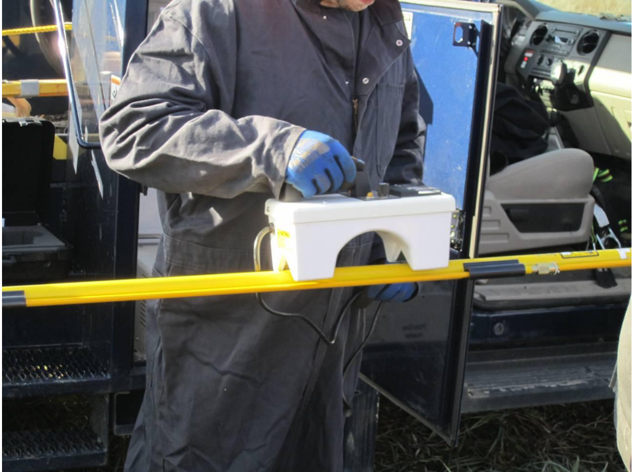
Figure 4-20 Lineman tests hotstick prior to installing the EPRI sensors on the energized 230 kV line
