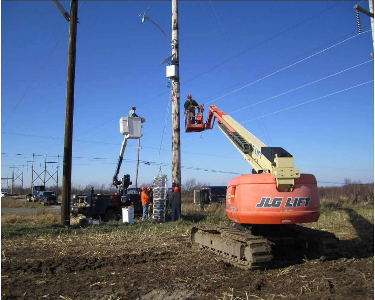
Figure 4-25 Solar panel for the ThermalRate system being rigged for installation
