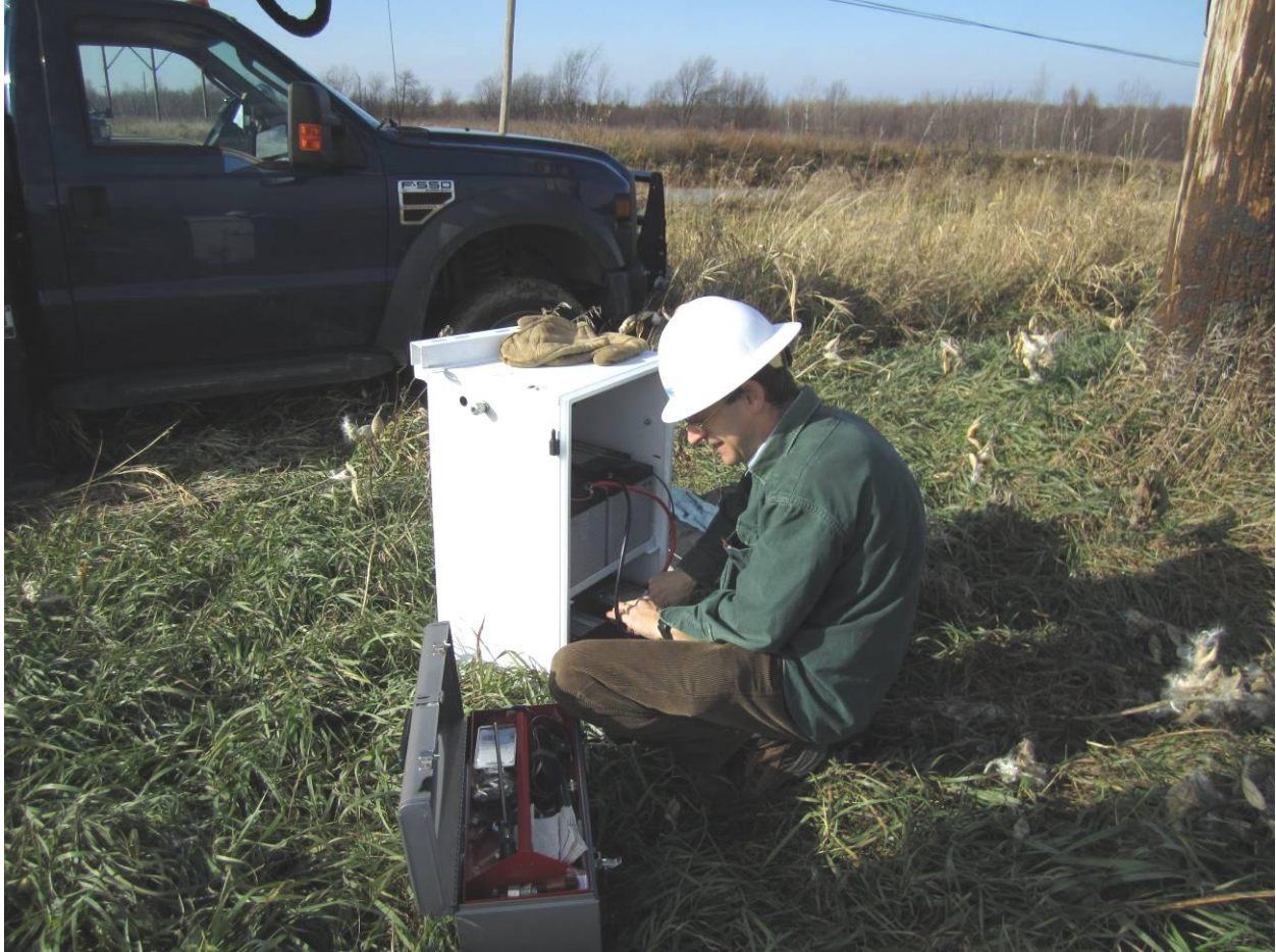
Figure 4-26 ThermalRate Battery Box being wired
