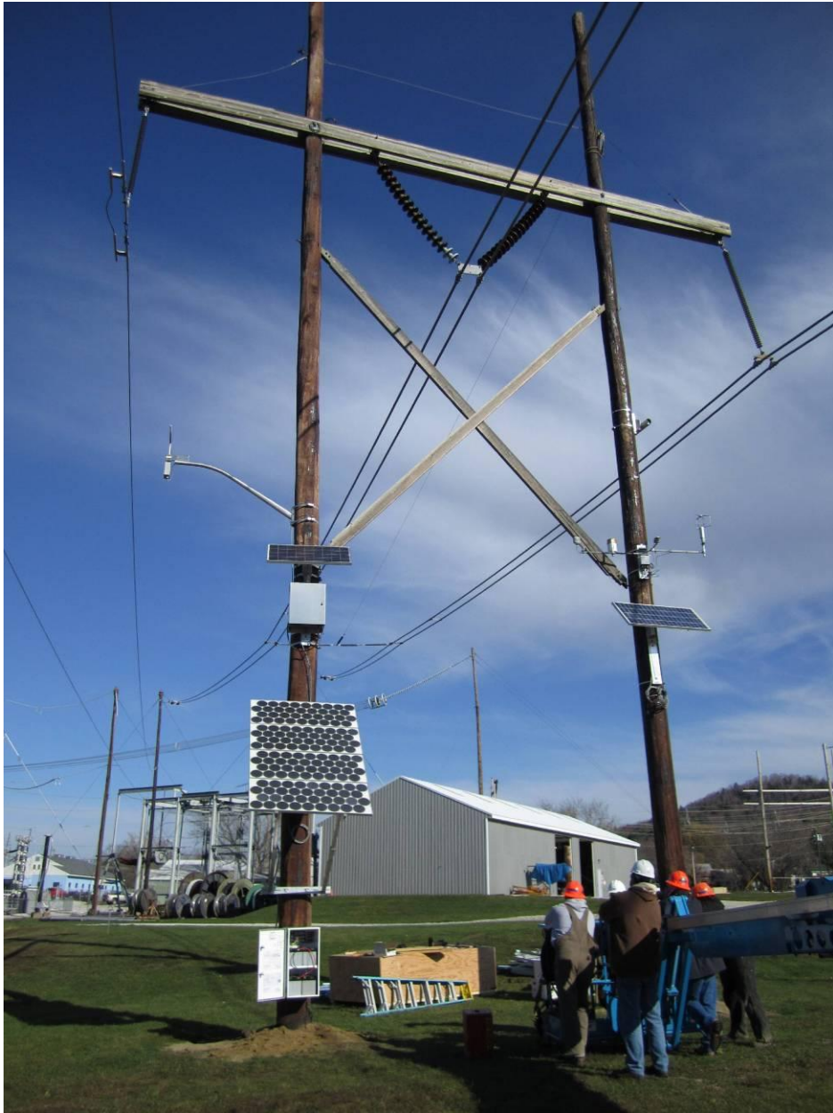
Figure 4-14 Near completion of the practice installation at EPRI Lenox.
