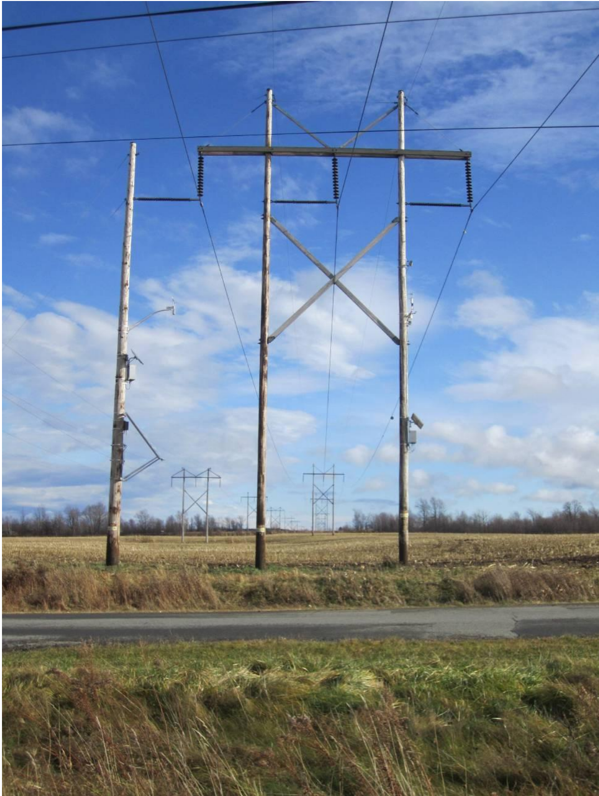
Figure 4-31 WP2-01/02 – “Site 1” completed - looking in an easterly direction
