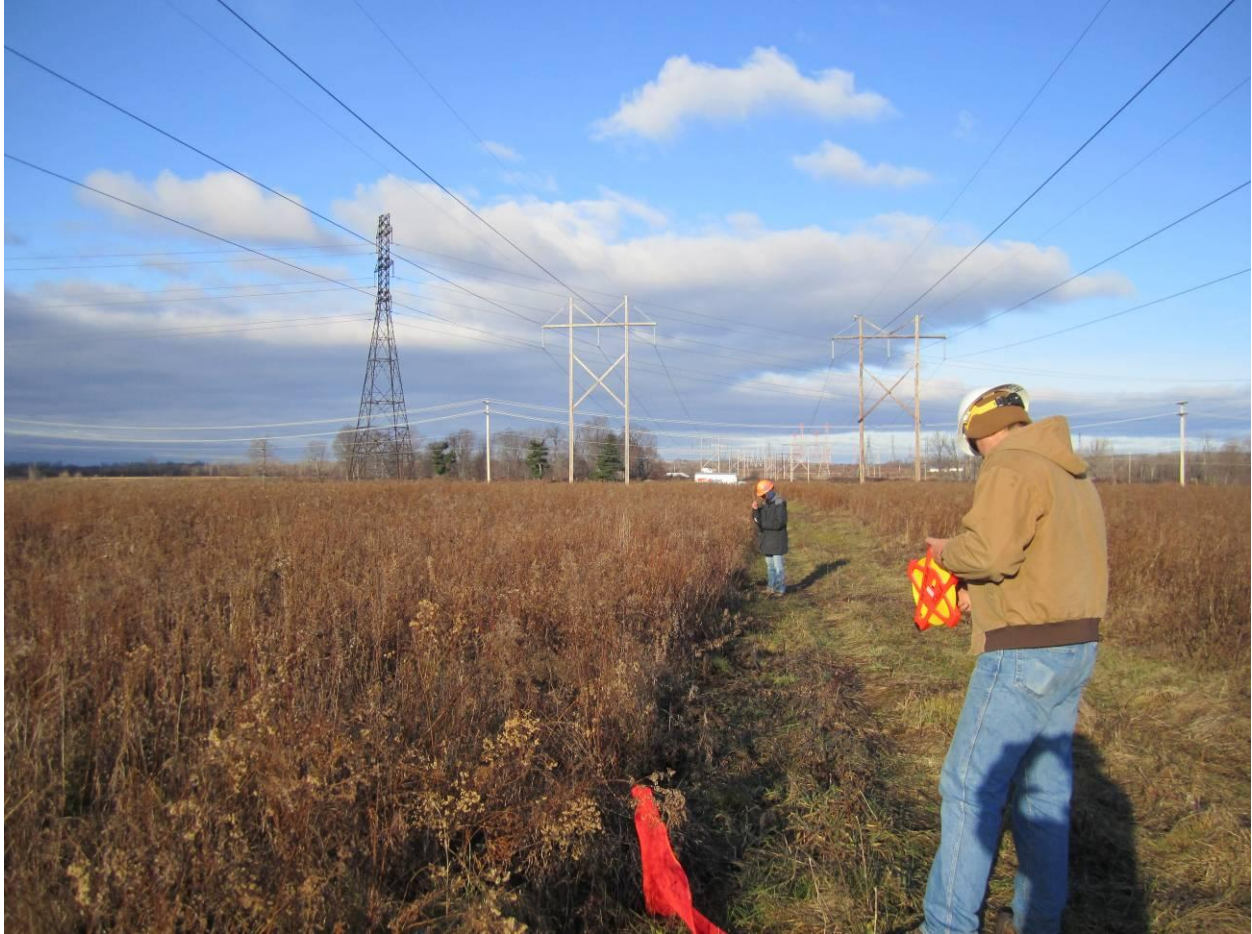
Figure 4-57 Locations were marked under the line for the sagometer target and EPRI sensors
