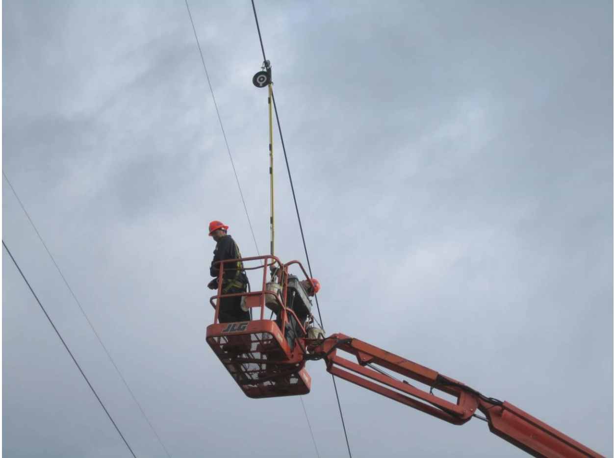
Figure 4-47 Installing the Sagometer target
