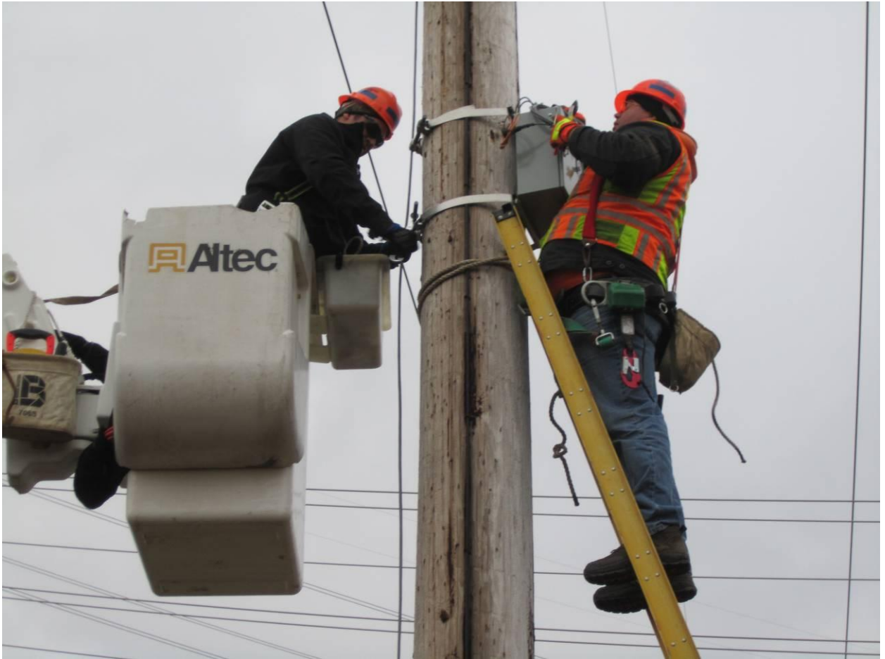
Figure 4-62 Linemen install ThermalRate electronics box
