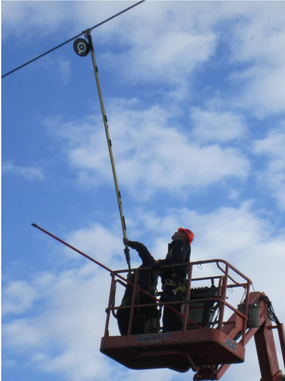
Figure 4-29 Sagometer target being installed
