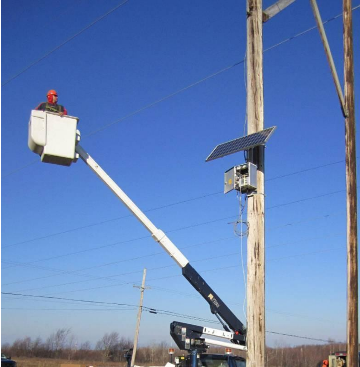
Figure 4-30 Sagometer electronics box and solar panel being checked after installation
