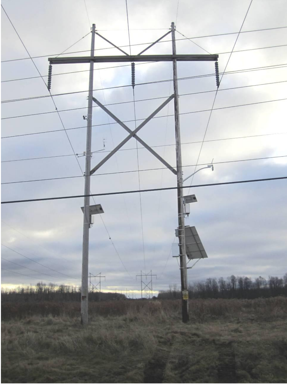
Figure 4-68 MW2 03/06 site completed looking back in the direction of Willis Substation
