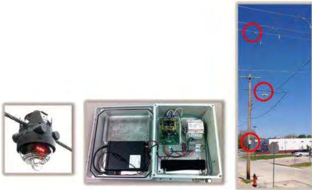
Figure 2-57: Typical Recloser Installation
