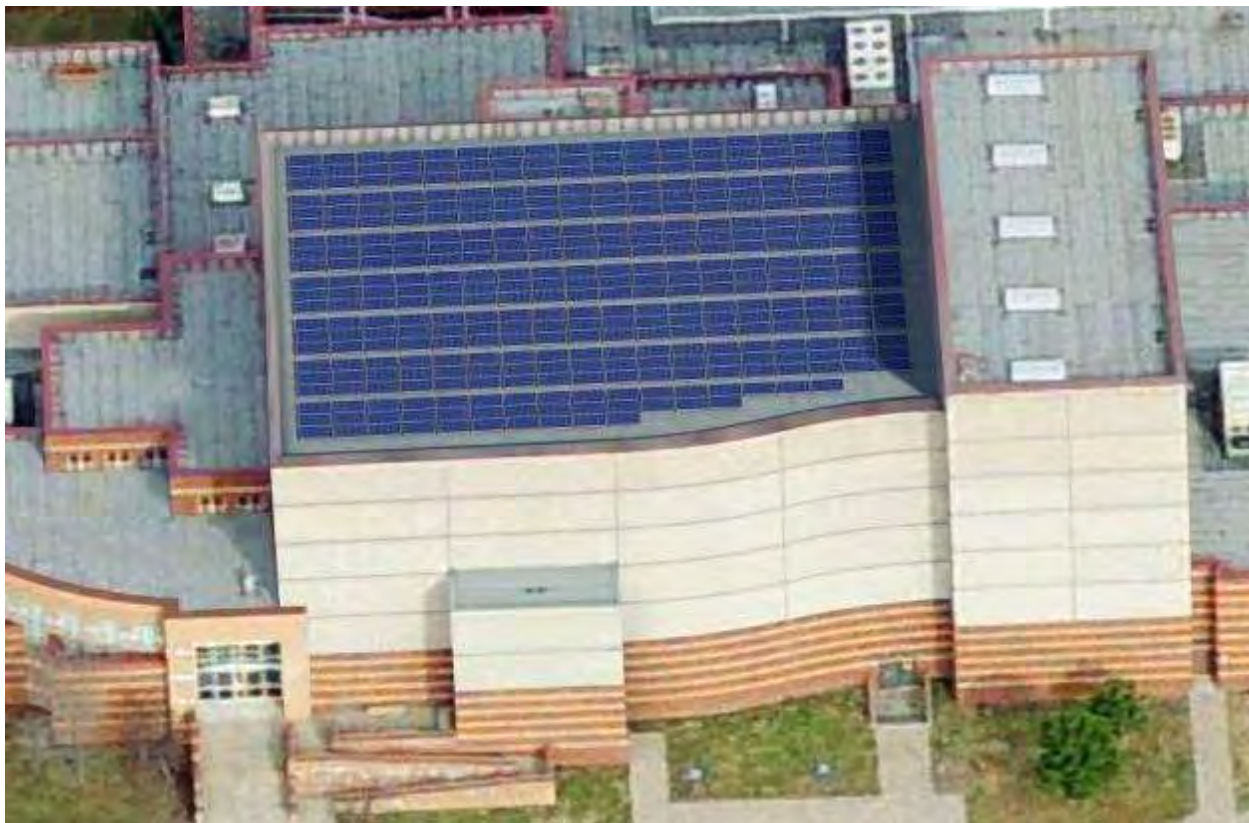
Figure 1-28: Paseo High School Roof-top Solar PV System
