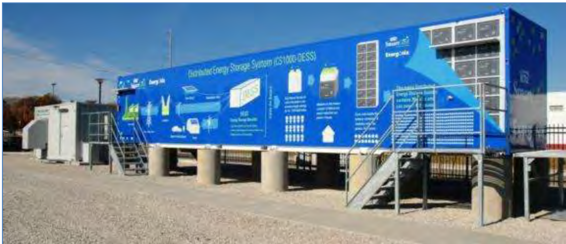
Figure 1-27: Grid-Connected Battery
