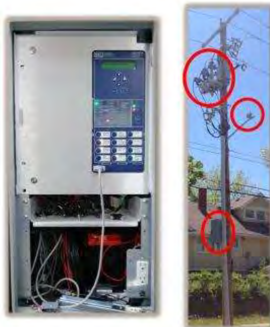
Figure 2-57: Typical Recloser Installation
