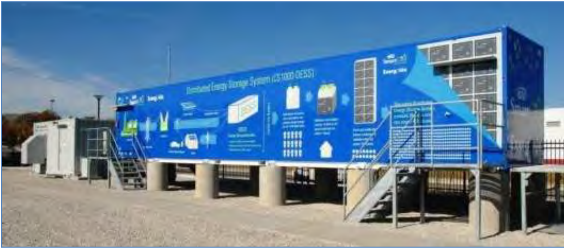
Figure 2-65: BESS Installation
