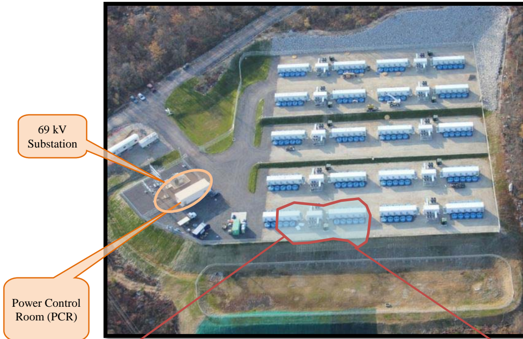
Figure 1 - Overview of plant, in Hazle, PA, with 200 flywheels (20MW capacity)
