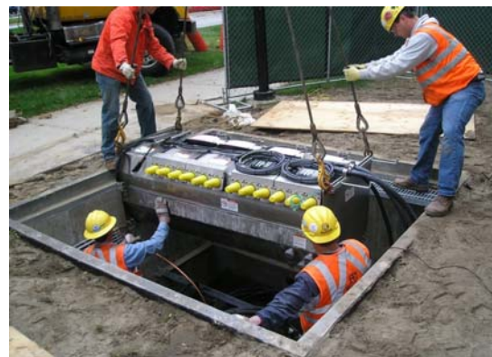
Figure 3.17: Installation of underground HRDS switch
