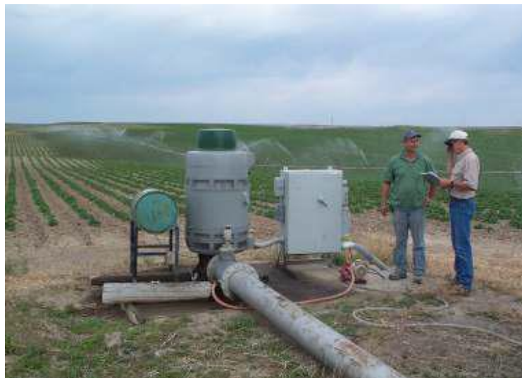
Field Installation of an Irrigation Load Control Package at Idaho Power Company
