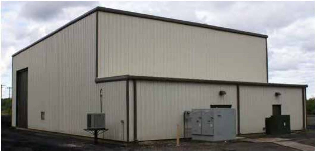
Figure 8 Ashlawn Battery Building, Painesville Municipal Electric Power, 325 Richmond St., Painesville, OH 44077.
