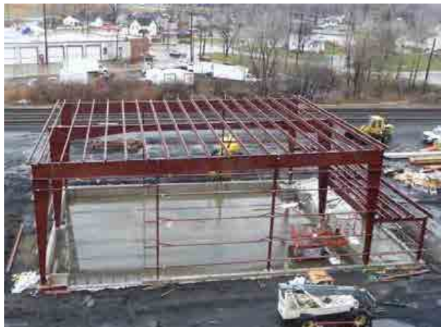
Figure 38 Painesville Battery Building during Construction.
