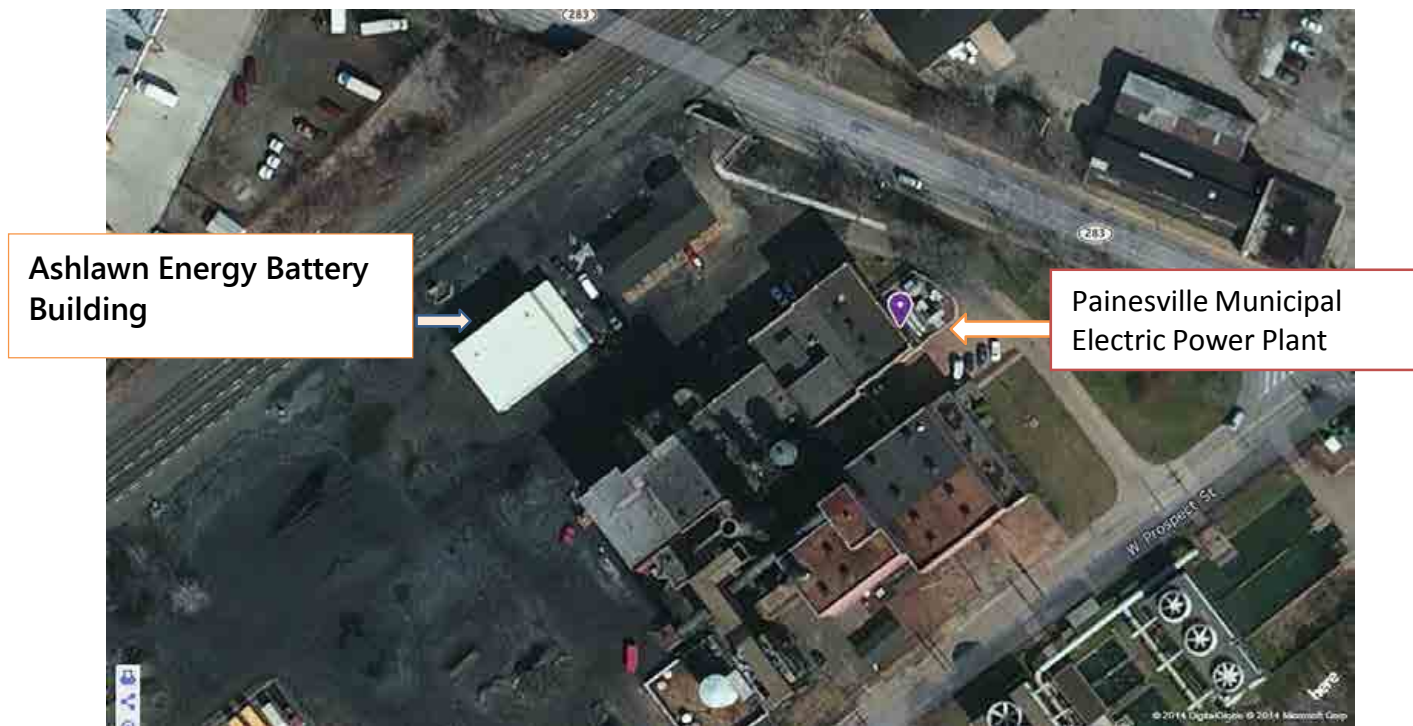
Figure 7 Painesville Municipal Power and Battery Building, 325 Richmond Street, Painesville, OH 44077.
