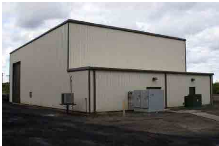
Figure 39 Completed Battery Building in Painesville, Ohio.
