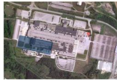
Full Scale Manufacturing in Westmoreland PA ~300,000 sf
