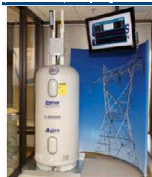
Figure 13.7: Typical Example of a GETS System Integrated with a 105-Gallon Marathon Hot Water Heater, on display at the PJM RTO (courtesy of Steffes Corporation)
