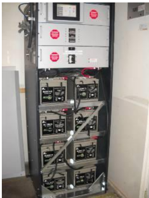
Figure 13.2: 9-kW SP Unit with Cover Removed
